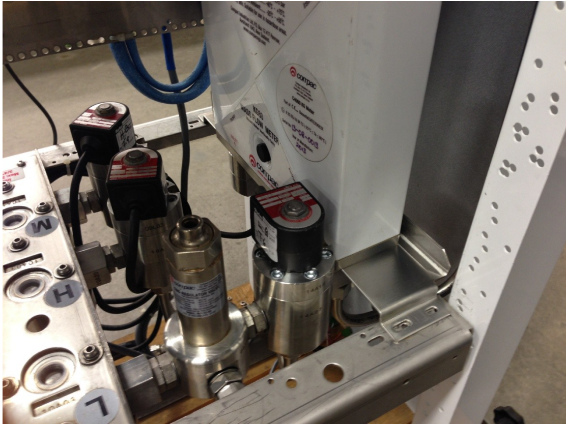
Installed meter prior to fastening to chassis.
