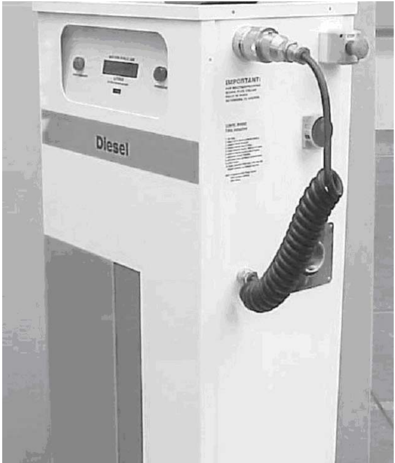
Electronic Over-fill Protection Cable and Connector
